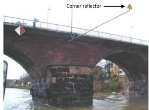
Figure 14 Corner reflector on a bridge
