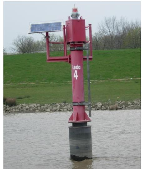
Figure 10 Steel beacon without radar reflector
