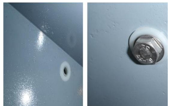
Figure 37 Plastic insulation between different metals
