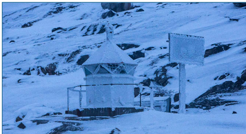
Figure 11 Example of ice on AtoN structure
