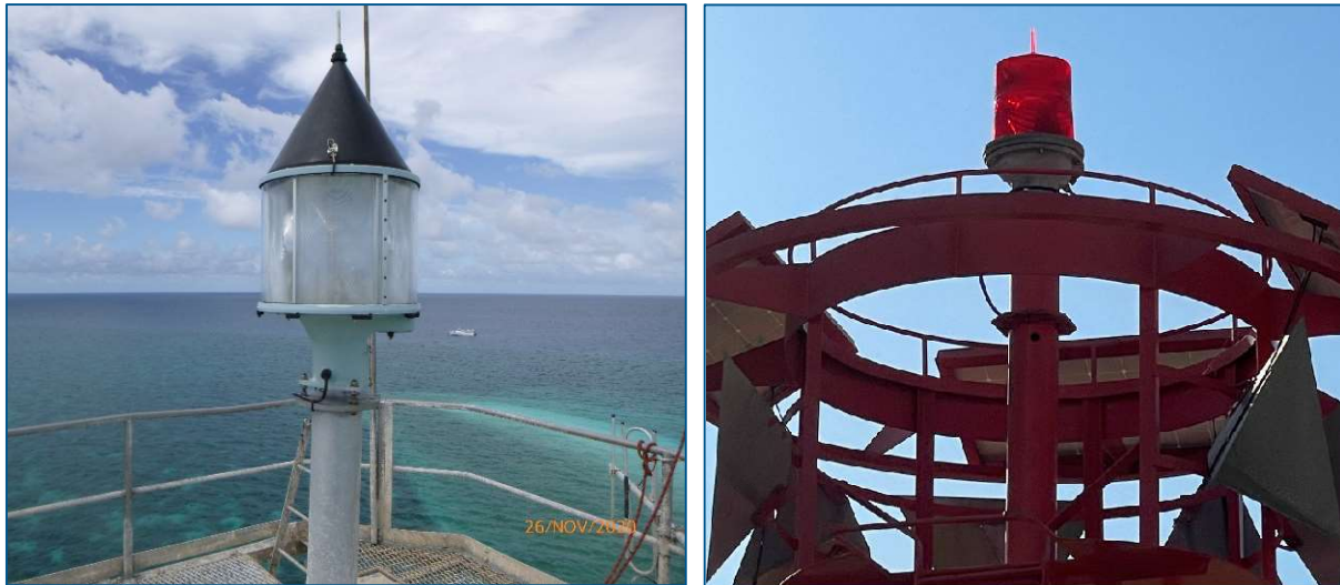
Figure 26 Example of AtoN configuration to deter bird roosting
