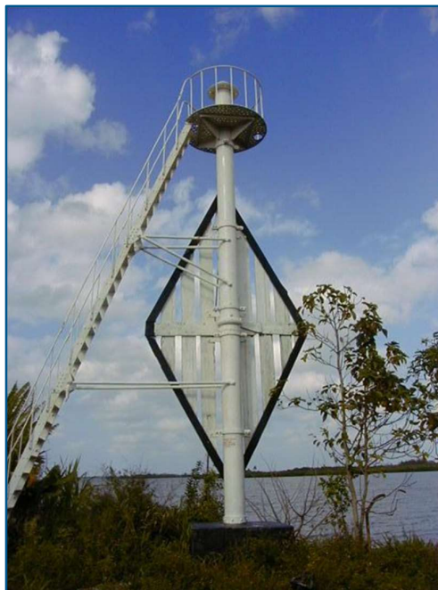
Figure 2 Front leading light with daymark lattice design
