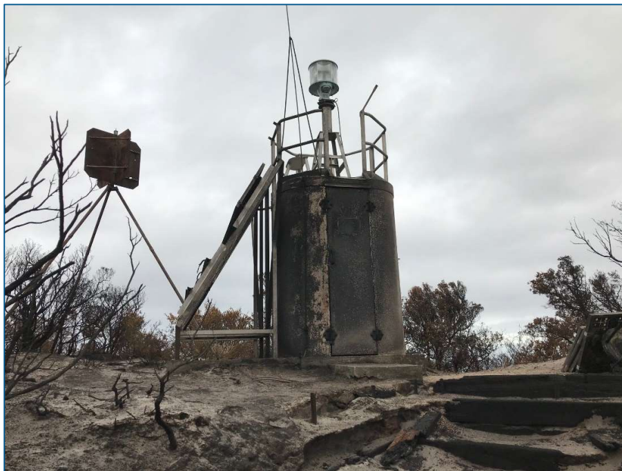
Figure 19 Example of AtoN destroyed by fire
