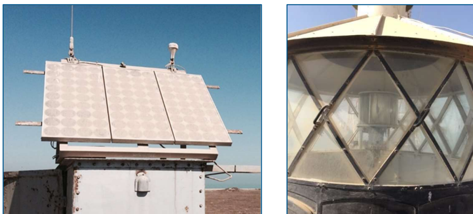
Figure 17 Presence of dust on AtoN device
