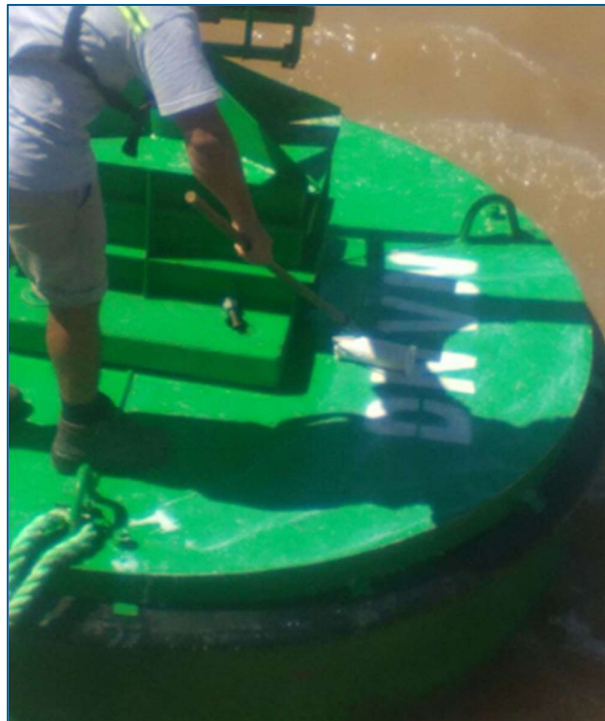
Figure 25 Anti-graffiti product application over the surface colour
